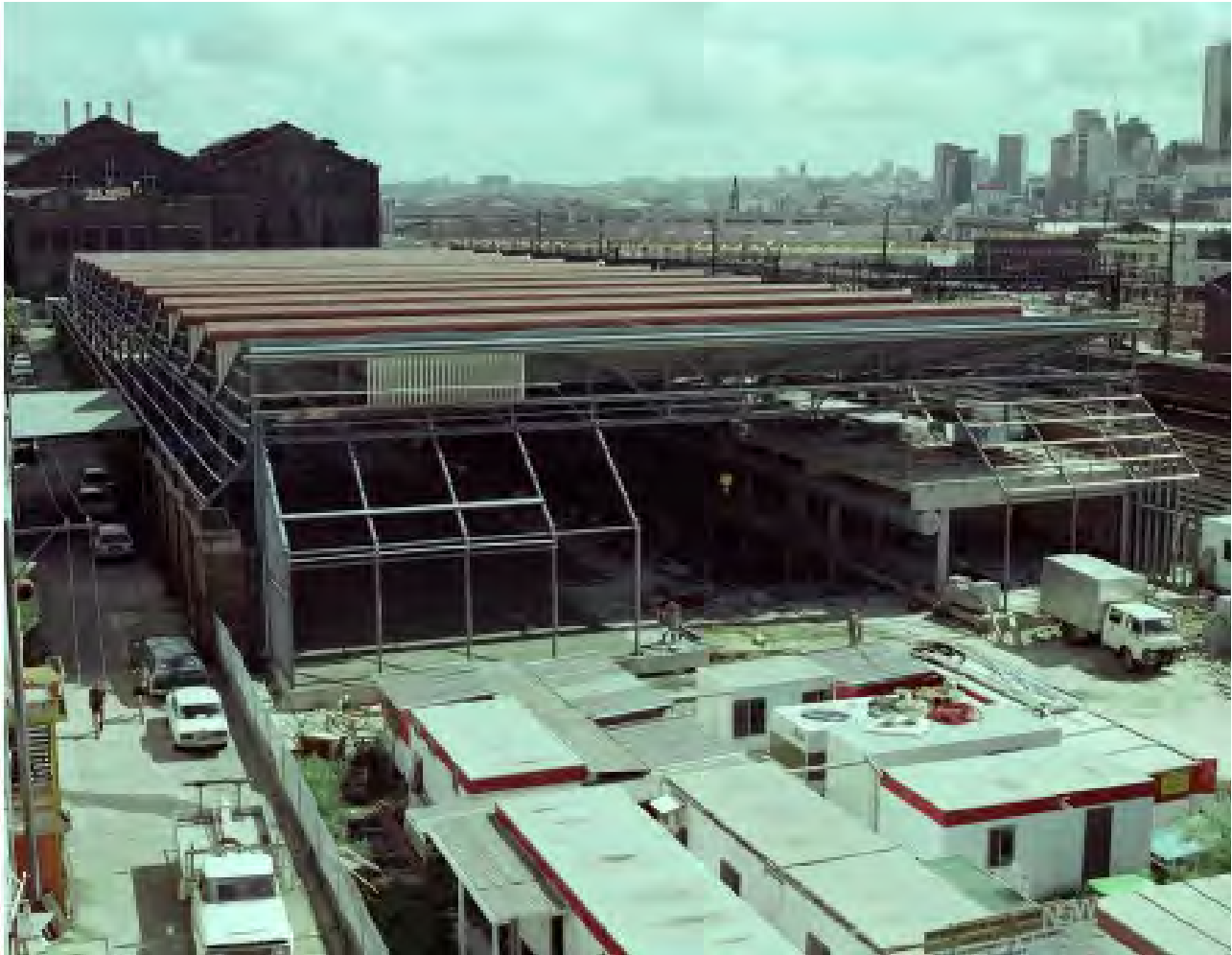
Figure 8 South elevation of the former Tram Depot (Harwood Building) during works, 1981
