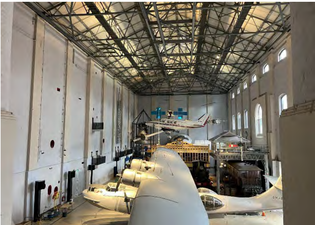
Figure 5 View from level 2 mezzanine of the Boiler House, looking north: the Catalina flying boat (foreground) had been lowered by February 2024
