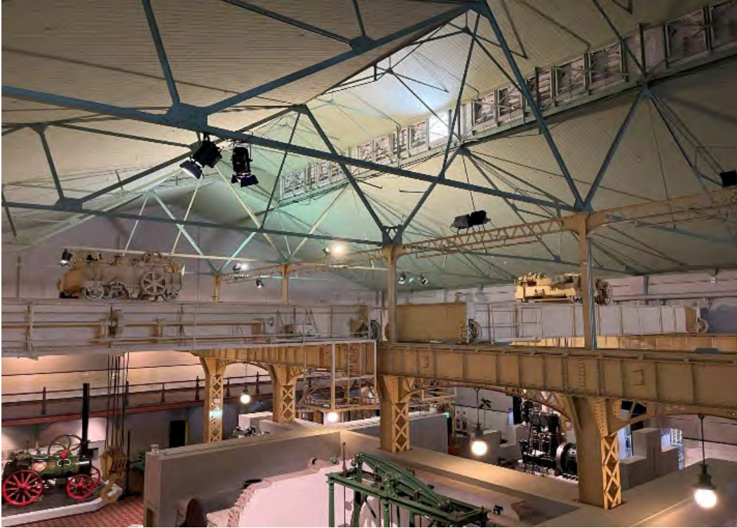
Figure 1 View of the Engine House from the bridge at level 3
