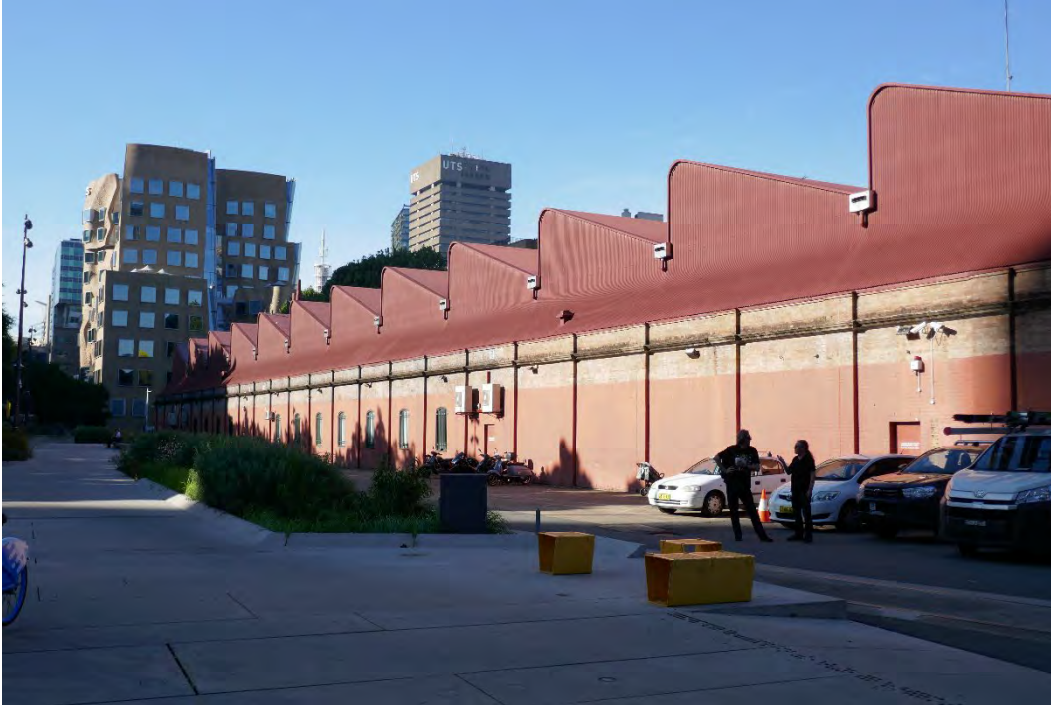
Figure 24 East elevation of the Harwood Building (part), looking south: the nine brick bays at the south date to 1899, and the roof form dates to 1981
