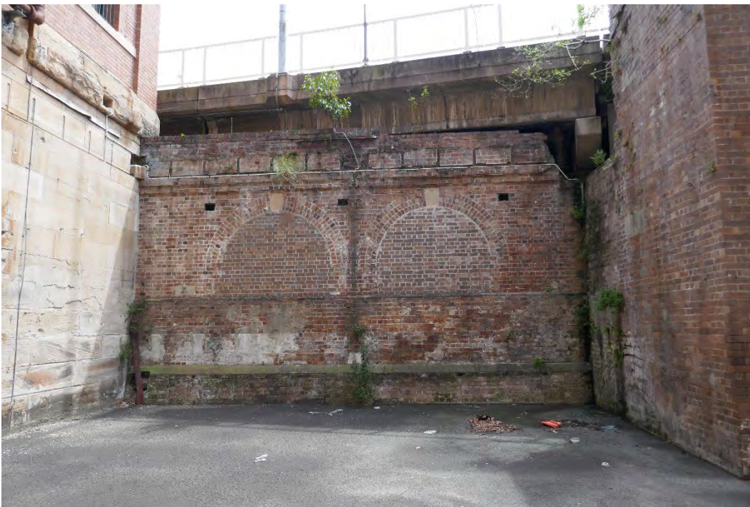
Figure 12 Arched openings, infilled, to the north of the former Pump House
