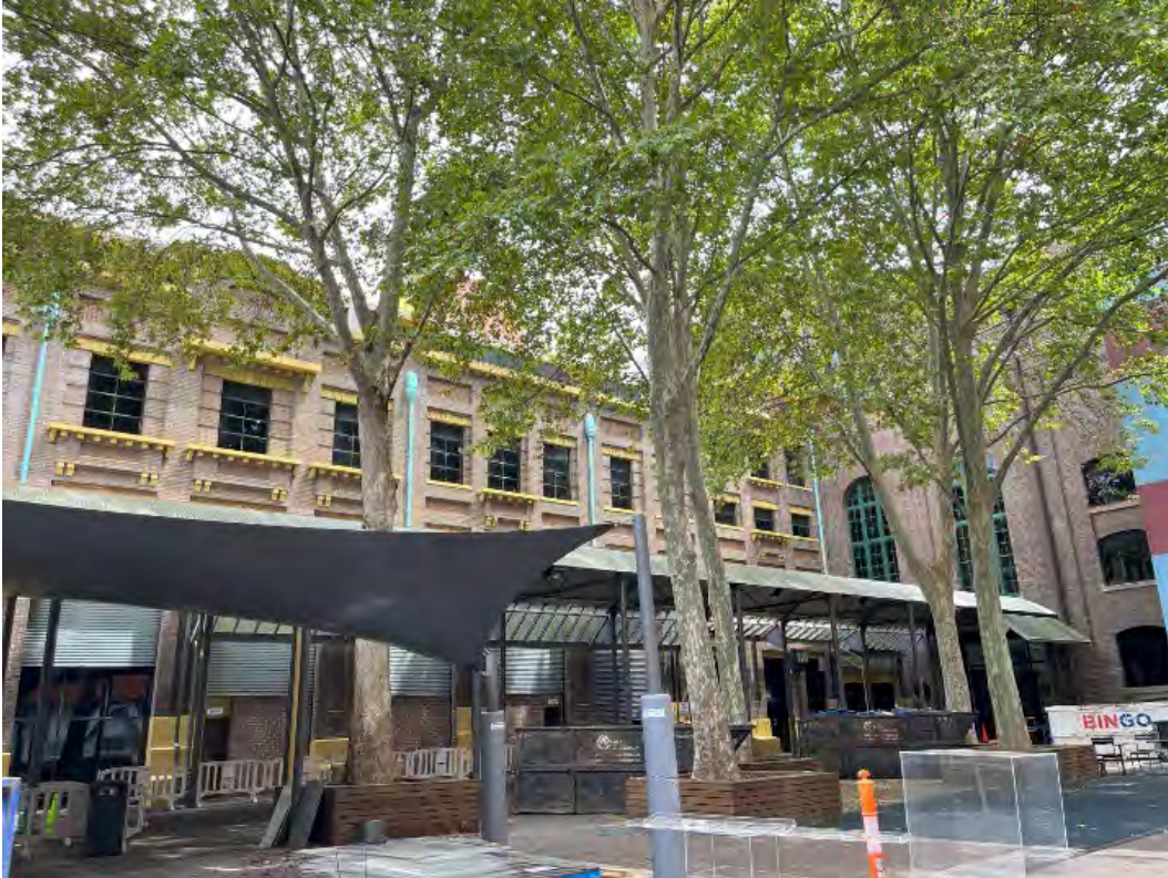
Figure 43 View from the Grace Bros Courtyard looking towards the Switch House
