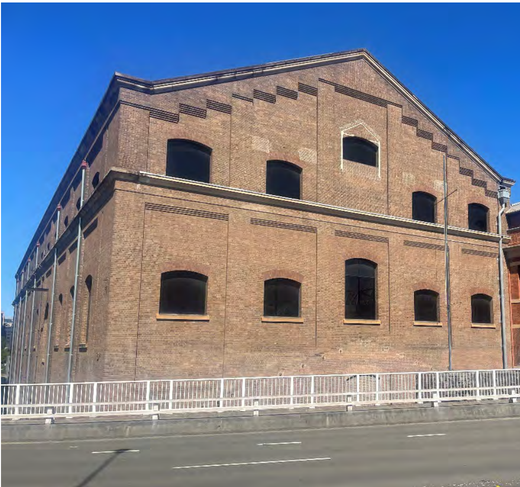
Figure 3 North and east (part) elevations of the Boiler House as seen from William Henry Street
