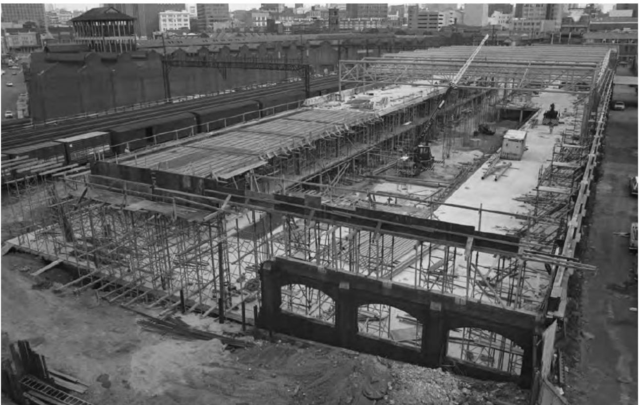
Figure 7 Works for the adaptive re-use of the Tram Depot underway, November 1980 Source: Powerhouse Museum Photo Library ST1D-SMN-16-12A
