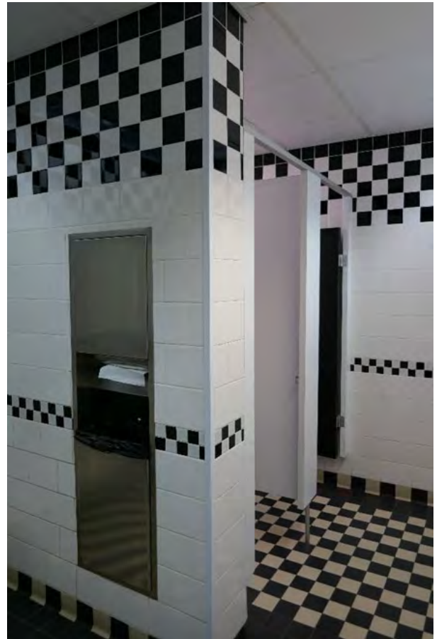
Figure 35 Bathrooms and wet areas are finished in black and white tiles throughout
