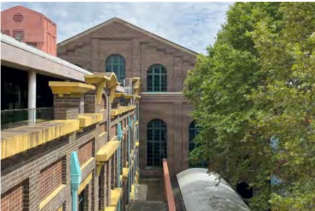
Figure 17 View of the Turbine Hall south elevation (part) from the Switch House (left)
