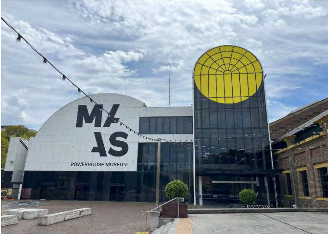
Figure 29 South elevation, February 2024
